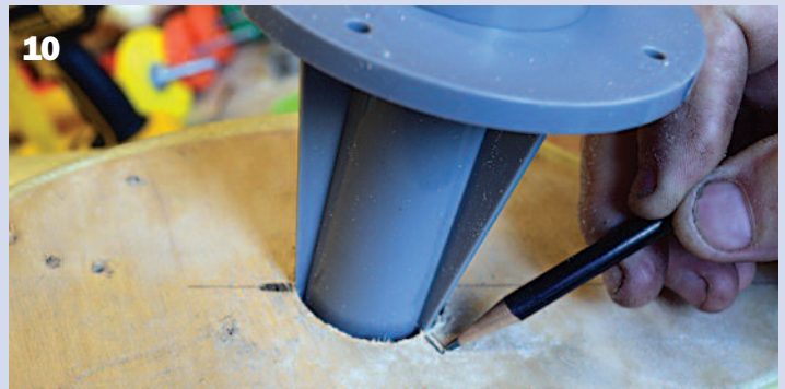
10. A dark pencil line is now drawn at the point of each stabilization wing.
